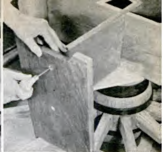
COUNTERBORE the legs about 1/8-in. deep to conceal the screw-head, finishing actual assembly
